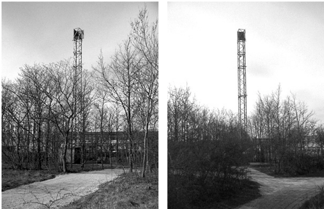
Figure 1.3: The lattice steel test mast seen from the east and north sides.
